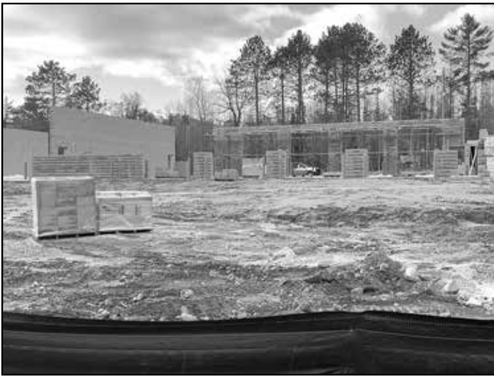
Auxiliary building under construction at Mercer Ranger Station. Photo Mike Hittle
