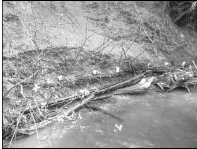
A fascine, or bundle of live cuttings, at the toe of an eroding bank.
